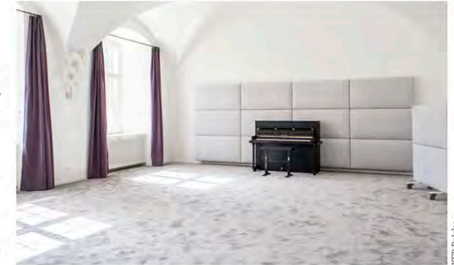
Above: To respect the protected architecture of Musikinsel Rheinau, acoustics have been improved through the use of carpet, curtains and radiator cladding, in addition to mobile and fixed panels
